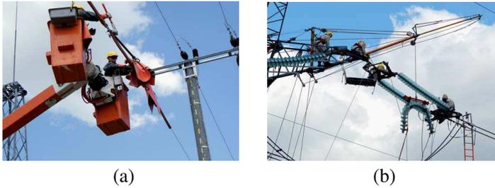
**Figure 1.** Live-line working on overhead lines. (a) Hot-glove workers on 15 kV line. (b) Hot-stick workers and bare-hand worker on 400 kV transmission line.
