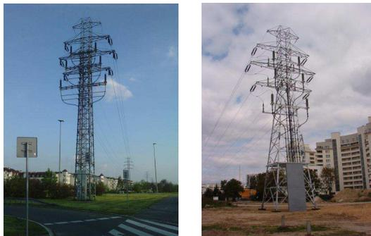
**Figure 1.** Transition towers of 110 kV overhead-underground transmission lines.
