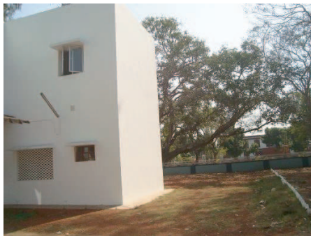
Figure 11. Photograph of measurement site.
