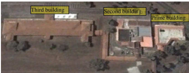
Figure 6. Test bay buildings.
