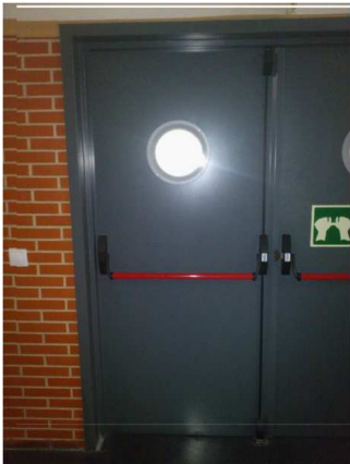
Figure 1. Metallic door with porthole window.
