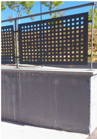
Figure 4. Metallic grid picture.
