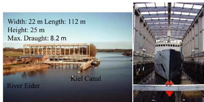
**Figure 10.** The EFS facility at Shirnau, Germany.
